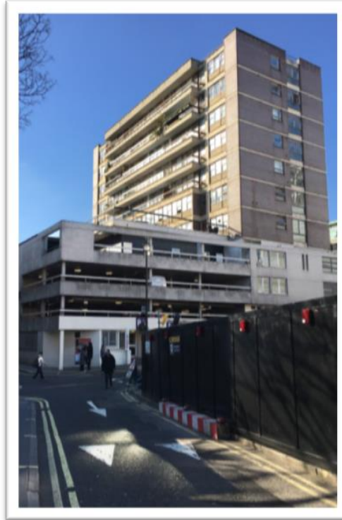
View 2: Whitcomb Street & Orange Street
